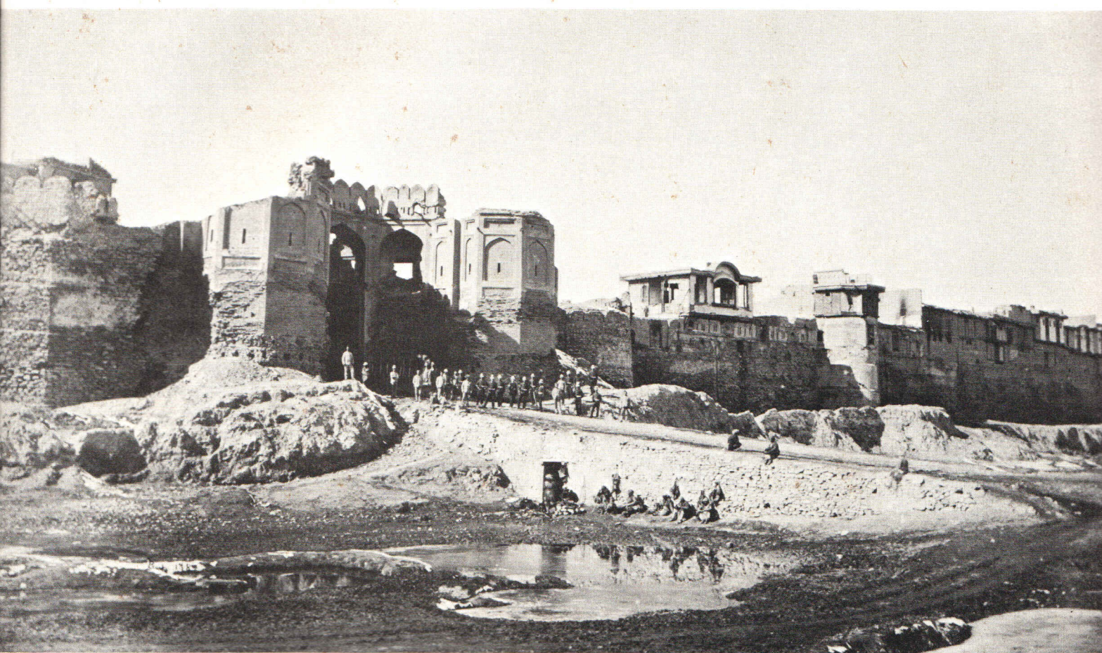
12-foot-thick walls, it dominated the city. General Roberts occupied it from the time he arrived until he set out on his long march to Kandahar.
